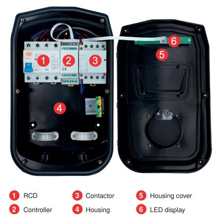
The charging station contains all the components required for controlling the charging process and for communication with the vehicle.
